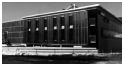
An Austrian hall and office building that uses solar for heating.
