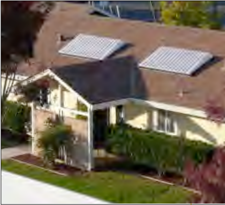
▲ Figure 1. Lakeland Electric, a Florida municipal utility, has SWH installed on customer roofs and then bills them for the energy over the life of the system as part of its utility services.
