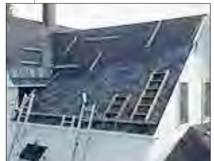
▲ Figure 1. Cleaning of the old shingle roof.
