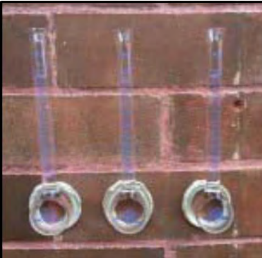
Masonry moisture testing
