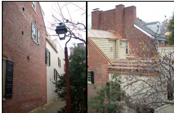
Precedent- 3 noisy neighboring air handlers
