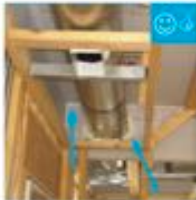
Seams and penetrations of air barrier properly sealed
