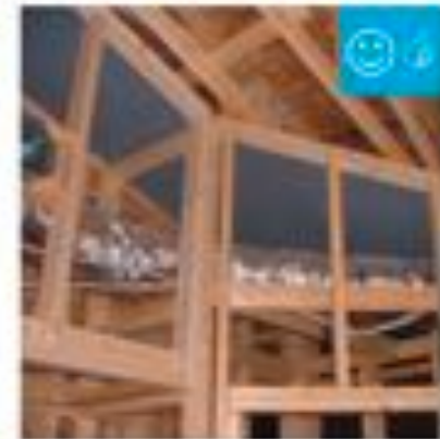
Air barrier is present between the dropped ceiling/soffit and the attic.
