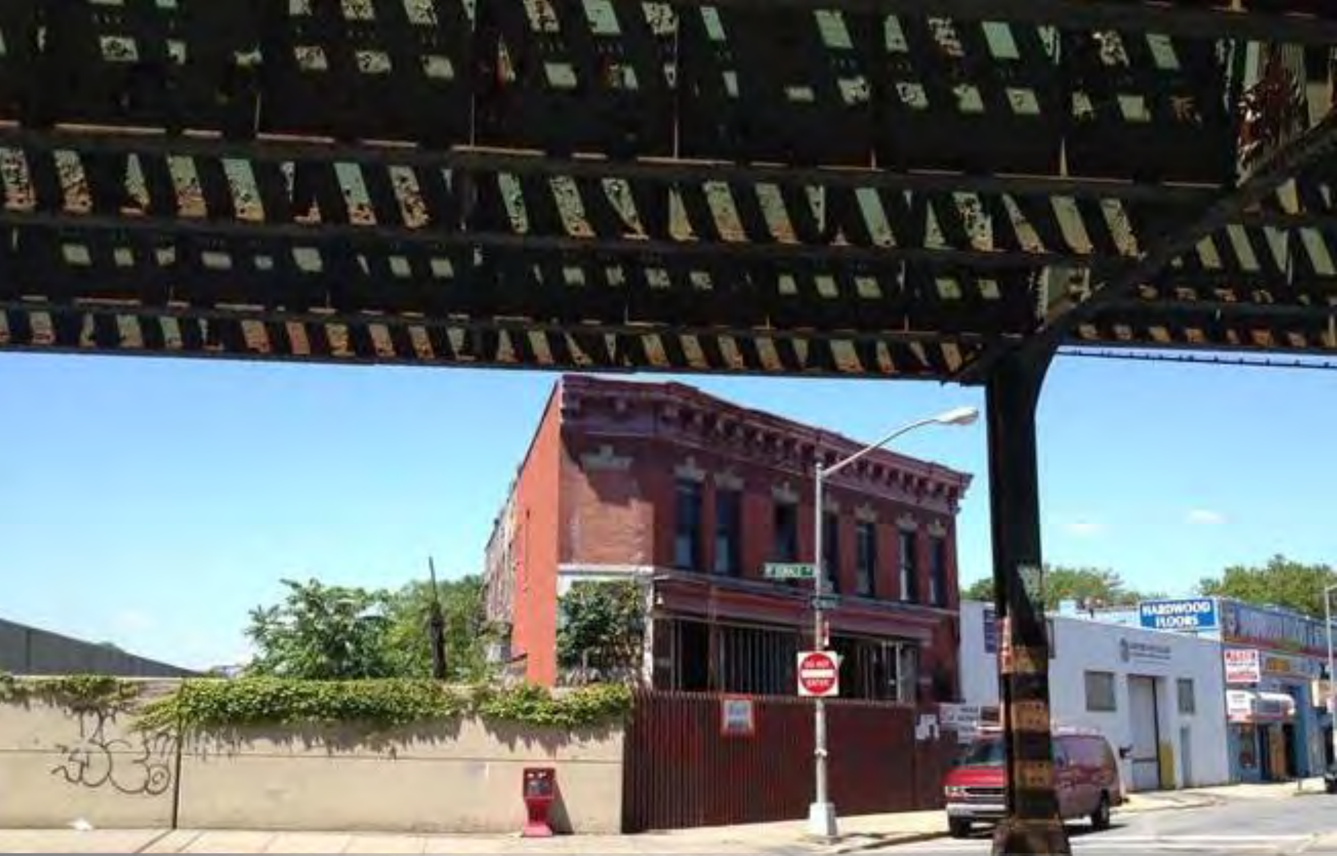
HATZOLAH CENTRAL AMBULANCE DISPATCH CALL CENTER Brooklyn, NY Alex E Romeo, Architect / Duncan Architect, CPHC
