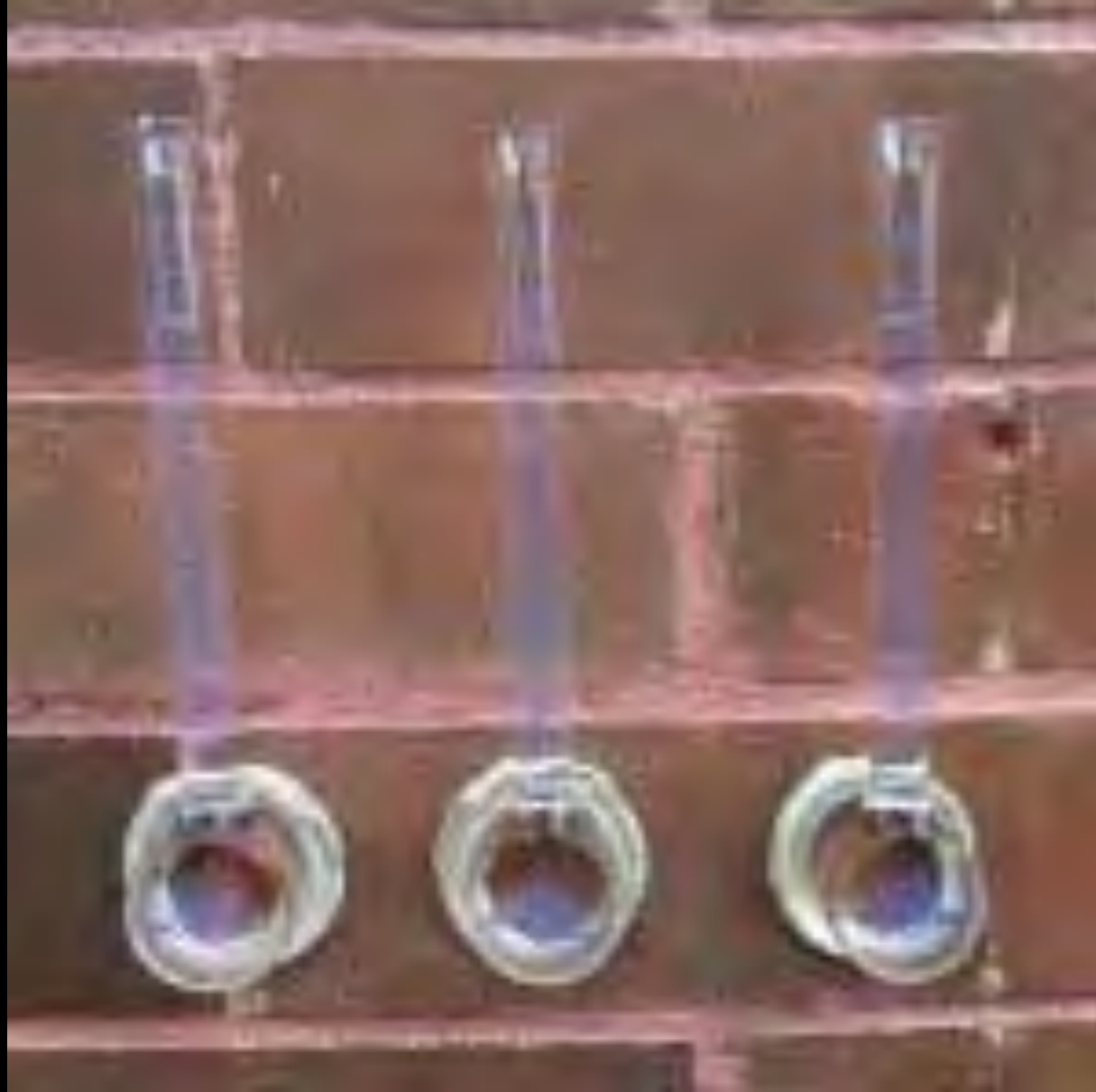
Masonry moisture testing
